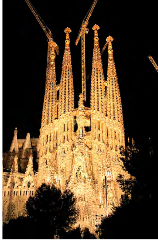
September 2011 Barcelona, Spain Desalination for the Environment
